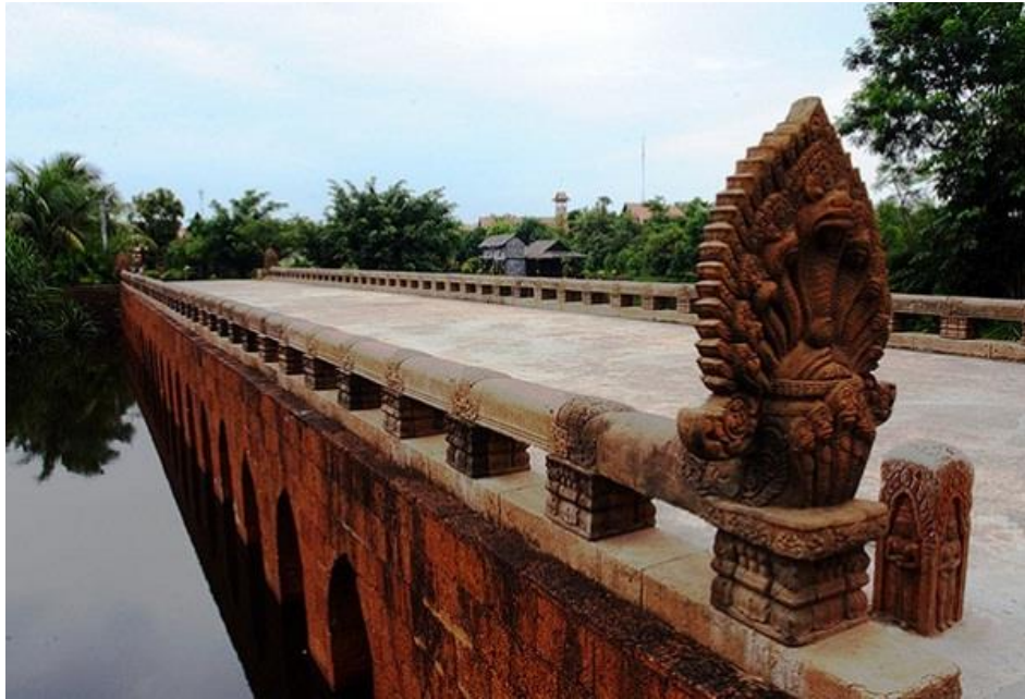
Kompong Krei Bridge, recognized as the longest corbelled stone ( https://goo.gl/images/2AsgXn )
